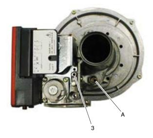
Check that the burner fan speed, corresponds to the data given in **table 5** of the "Technical gas data" booklet.
